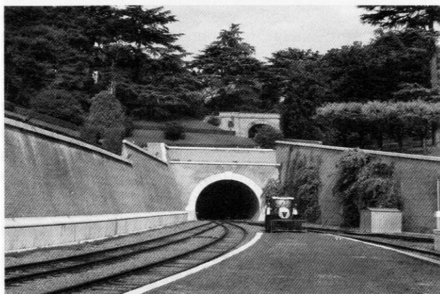
The headshunt tunnel at the end of Vatican City station platform
